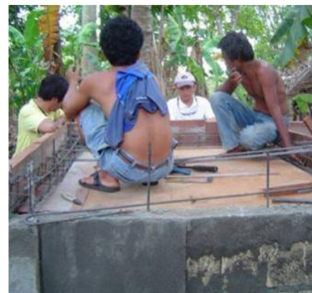
Figure 5: Construction of a UDDT (source: DILG-GTZ Program)
