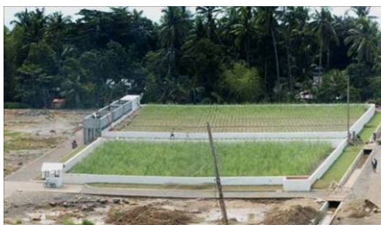
Figure 2: Constructed wetland (source: GEOPLAN Cebu)
