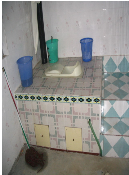
Figure 1: Domestic urine diverting toilet in Shaanxi Province (source: Plan China)
