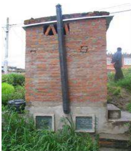
figure 1: Double vault urine diversion toilet (source: ENPHO)
